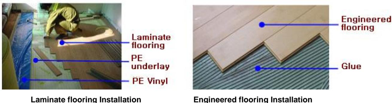
**Fig. 1.** Installation method of laminate flooring and engineered flooring
